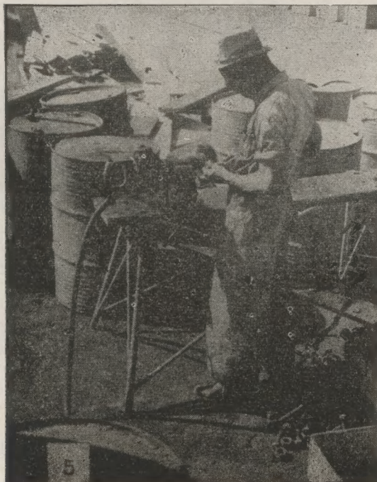
5 - Salvaging of bolts, which range in cost from a few cents to Fls. 5, is a continuous job. First they are cleaned with an electrically driven brush (which Epifano Vrolijk is operating in the photograph). The nut is removed, the threads are "chased" (thoroughly cleaned), alignment is checked, and the nut refitted.
